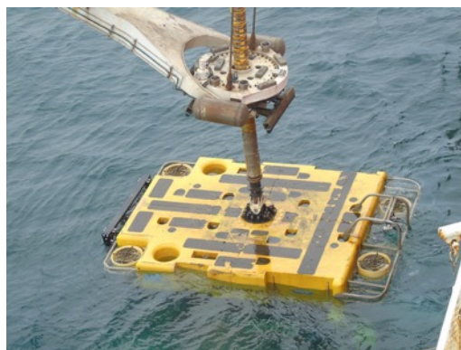
Sealion III working on Wando-Jinsan power cable PLIB (2017)
